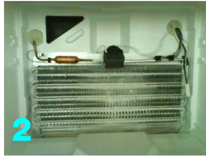
radiator kit replaced
